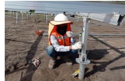
Mounting part installation
