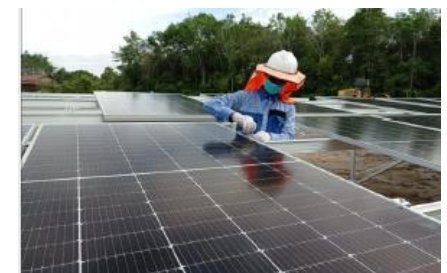
Solar panel installation
